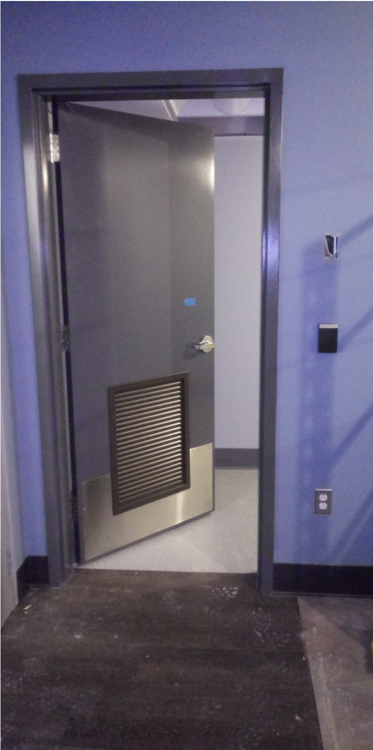
Dispatch 120 – Card reader installation continues thru out.
