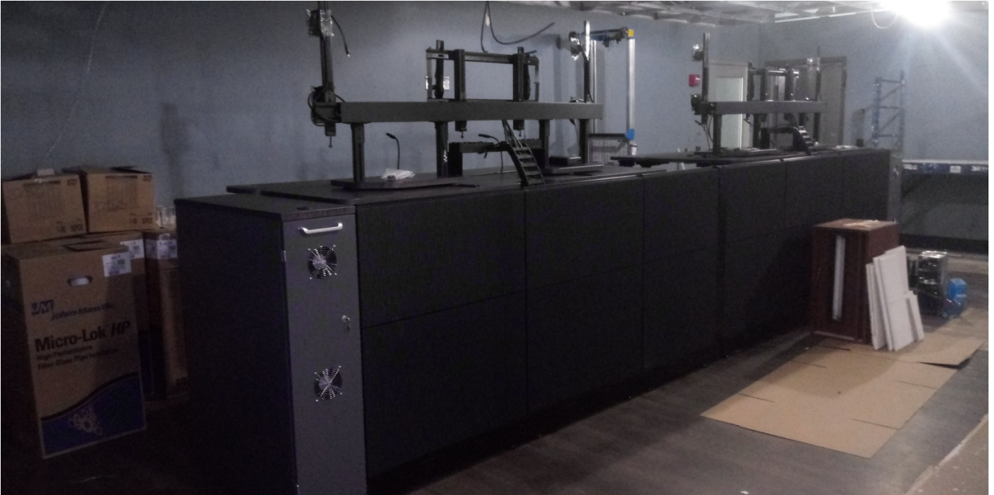
Dispatch 120 – Xybix Workstation installation continues.
