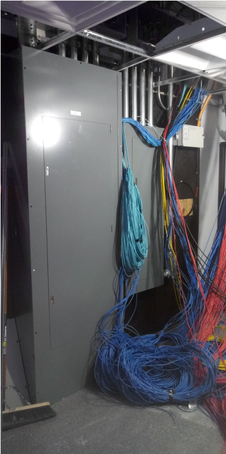
Server Room 122 – data wiring installations continue.
