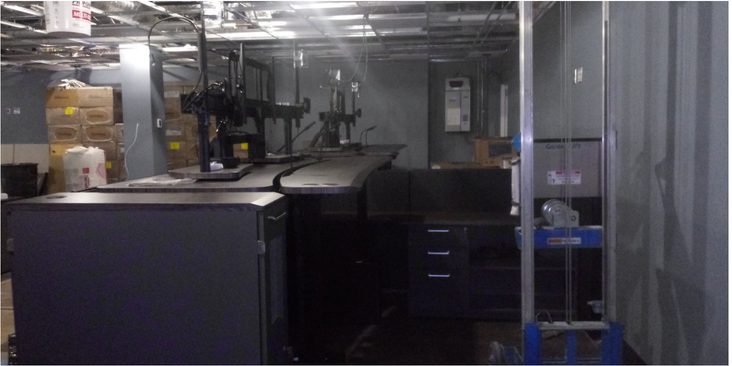
Dispatch 120 – Xybix Workstation installation continues.
